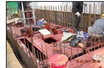
METAL FORMWORK
