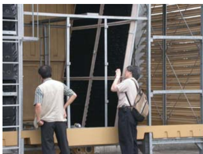
All visitors are very interesting to the construction of cooling tower.
